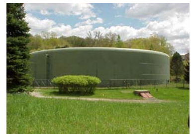
The Tarrywile Water Storage Tank
